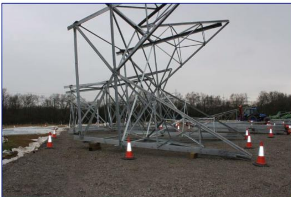
Image 4.5 Pylon steelwork preparation on the ground
