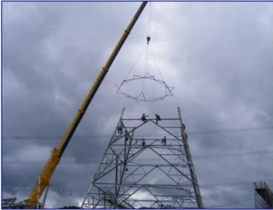
Image 4.6 Pylon erection
