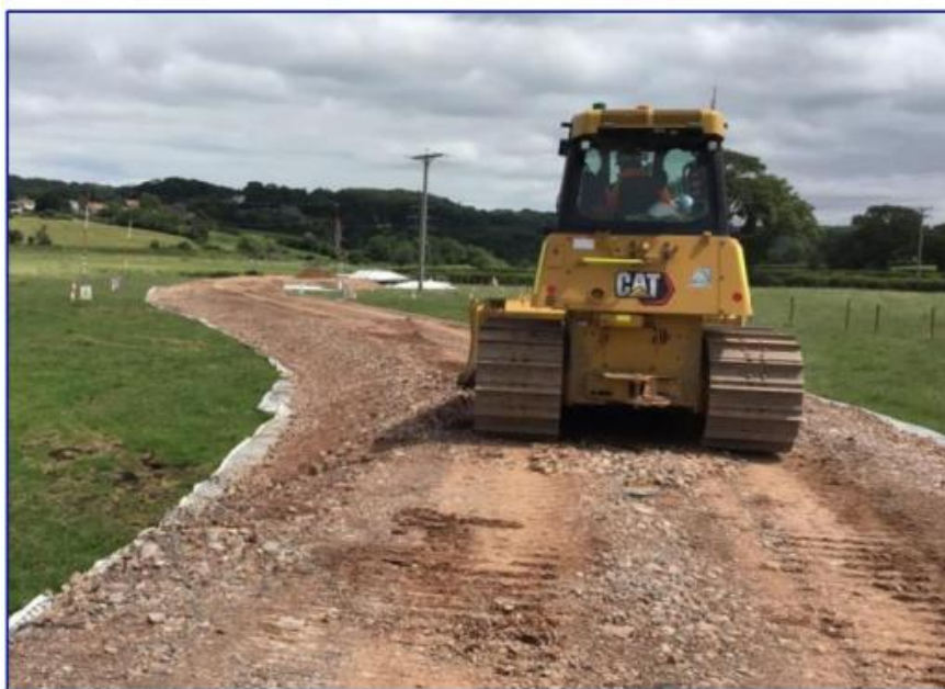
Image 4.3 Typical construction of a haul road
