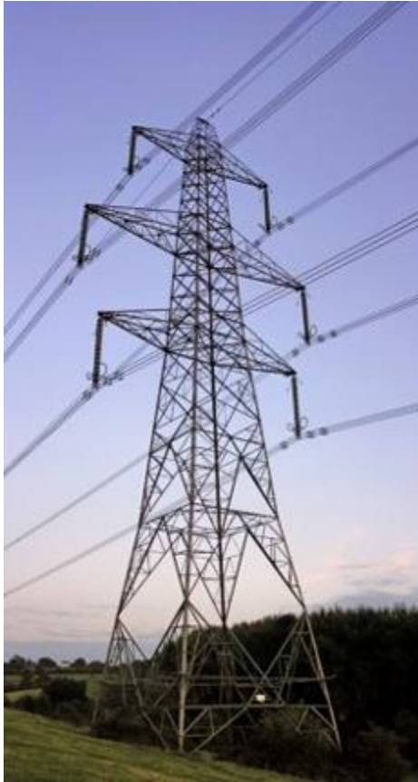
Image 4.15 Typical suspension steel lattice pylon 25
