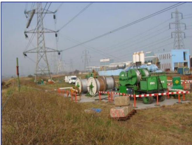
Image 4.7 Machinery associated with conductor pulling
